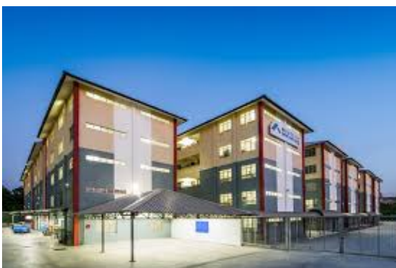
WESTLITE TAMPOI IN JOHOR
